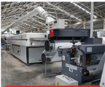
Extrusion Tape Line (Lohia Make)
